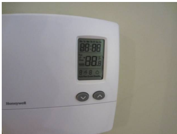
Error signs on thermostat display. Electric baseboard is not working adequately.
