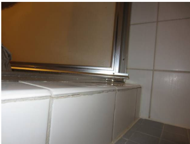
Cracked grout noted inside shower stall.
